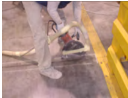
Inserimento tondino salva giunto Housing of the steel tendon-saving device
